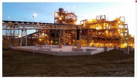
Industry Mining Commence June 2016 Complete July 2016 Region Ravensthorpe,WA Type of Work Demolition Dewatering Earthworks Concrete Repairs Formwork Concrete Reinforcement
